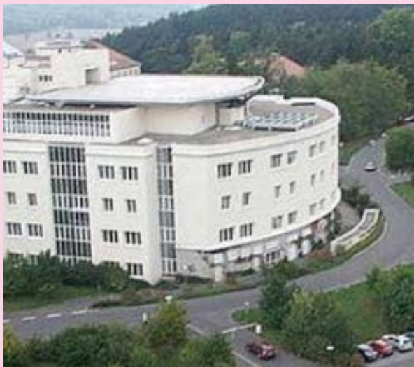
Figure 5 The Hospital at Bad Berka, with the Molten Carbonate Fuel Cell has been operational for 49,025 hours.
